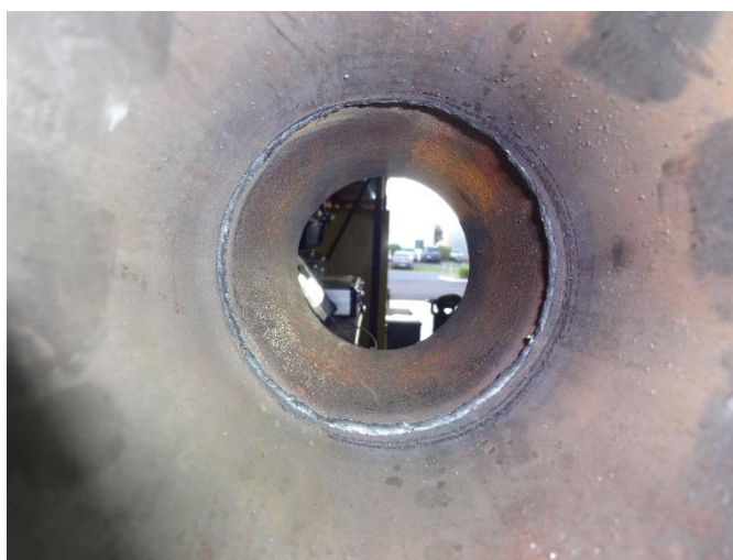
Typical View of Pipe Penetration
